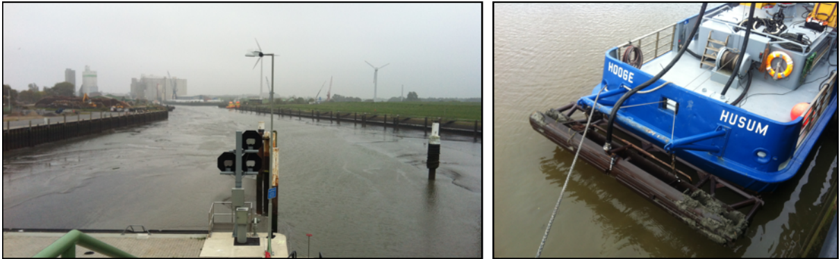
Figure 9: View at the mud shoals in the Port of Husum at low tide / Bed leveller used for mud conditioning
