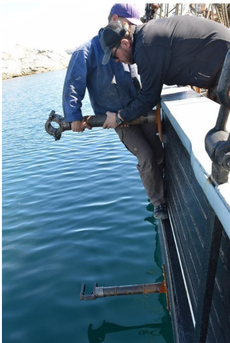
Figure 3: installation of transducer pole
